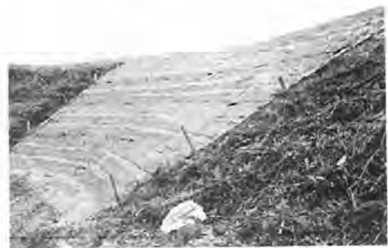
図9 盛立て完了 Completed Filling Work
