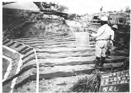
図8 GHDを用いた盛立て状況 Filling Work with GHD
