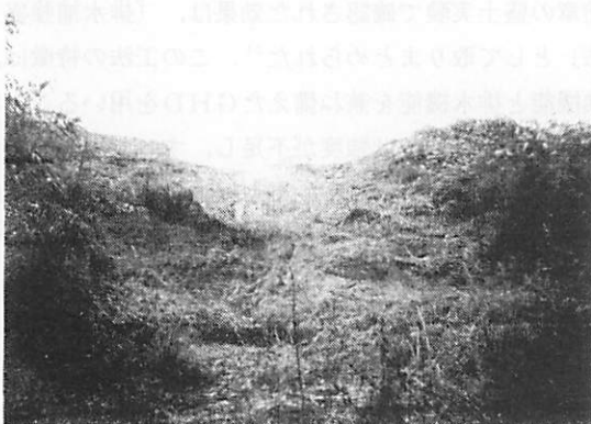
図7 崩壊斜面 Failed Slope
